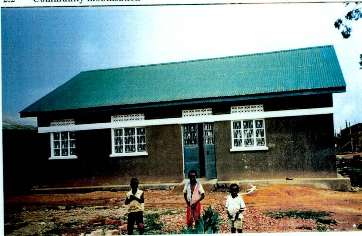
Completed Community Facility
